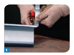
To trim a short piece of steel to length is a straight forward 'cut and peel'. Remember it's the off-cut that gets peeled away as you cut. Make sure you dispose of the off-cut appropriately or better still, recycle it!
