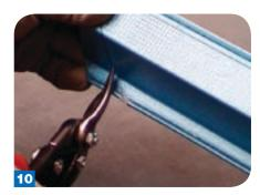
To **mitre cut** a roof batten, use a template or ruler to draw a guide. And like cutting C-studs, cut in at an angle to free up the lip material.
