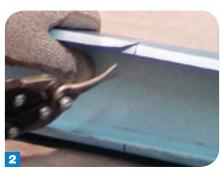
To cut a **C-stud section**, start by cutting an angle on the lip with either snip. This frees up material on the lip...
