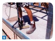
'Quik-Drive Pro' stand-up extensions fix timber or fibreboard to steel frames easily and efficiently.
