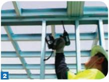
Regardless of the position or height of the job, an impact driver fixes quickly with minimum exertion – the tool's impact feature does most of the hard work for you.
