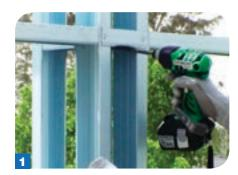
When using lithium battery impact drivers, easily access C-channel recesses by snapping on an extended hex insert bit.
