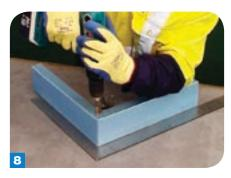
With the C-clamp holding the angle in place, fasten the two overlapping tabs.
