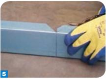
Using your snips, cut along the lines, snipping out all the pieces that need to be removed. Be careful not to cut off the tabs.
