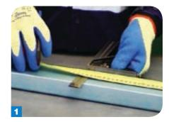
Measure out where you want to create your joint. In this example, we've measured 400mm from the end of the steel.
