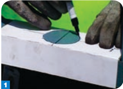
1 Mark the position of the hole with a ruler and/ or template.
