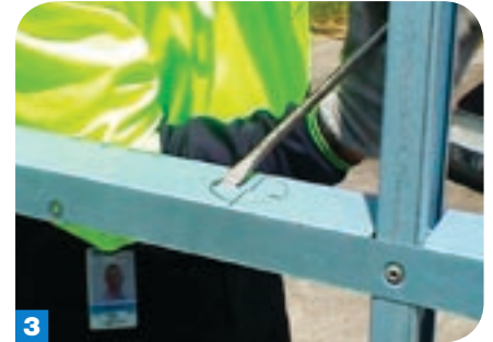
3 Use a screwdriver to open an entry point for the snips, and then, cut out with either your left-cut or right-cut snips.
