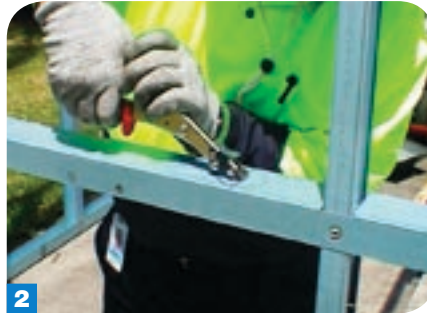
2 Before you use your snips, use pipe and duct snips (shown in the diagram) or a carborundum cutter to cut across the diameter of the hole. This will free up the material.
