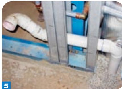
**5** Drilling **back-to-back C-channels** is simple.
