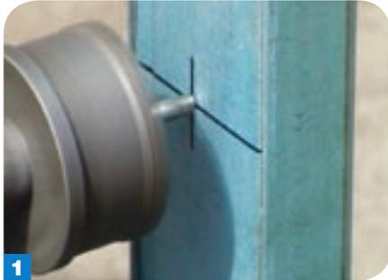
**1** To drill a penetration hole in a **boxed stud** first locate the centre point for the hole on one side of the stud and drill.
