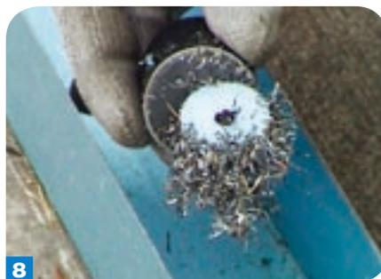
**8** Hole cutting creates swarf. Remove swarf to avoid risk of corrosion. For a professional result, clean up any swarf on the surface of the metal. Use a magnet to efficiently remove swarf from the base plate.
