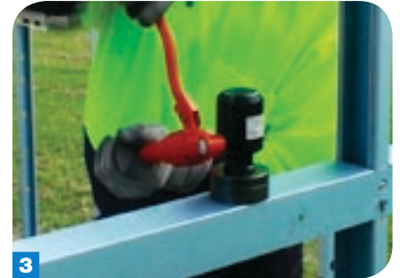
3 Use the punch for single C-channel studs, noggins and top plates.
