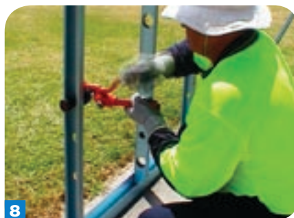
8 Or use the pre-made service holes already provided in the frame studs as pilot holes for the large punch.
