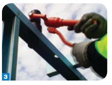
A manual hydraulic punch can be used for single C-channel stud, noggins and top plates. A swivel head and handle gives the operator access to studs or noggins from the side, or when working overhead on top plates.
