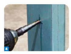
A pilot hole can be made with a clear-cut drill if working with light thickness steel, or with a half-inch step drill for thicker materials. Remember to use a lubricant to improve the cutting efficiency and increase the lifespan of your step drill.
